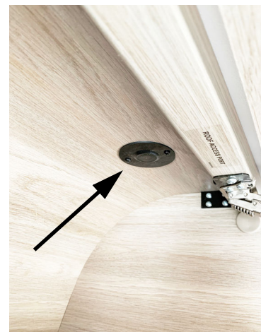
Roof Access Port -Typical View
